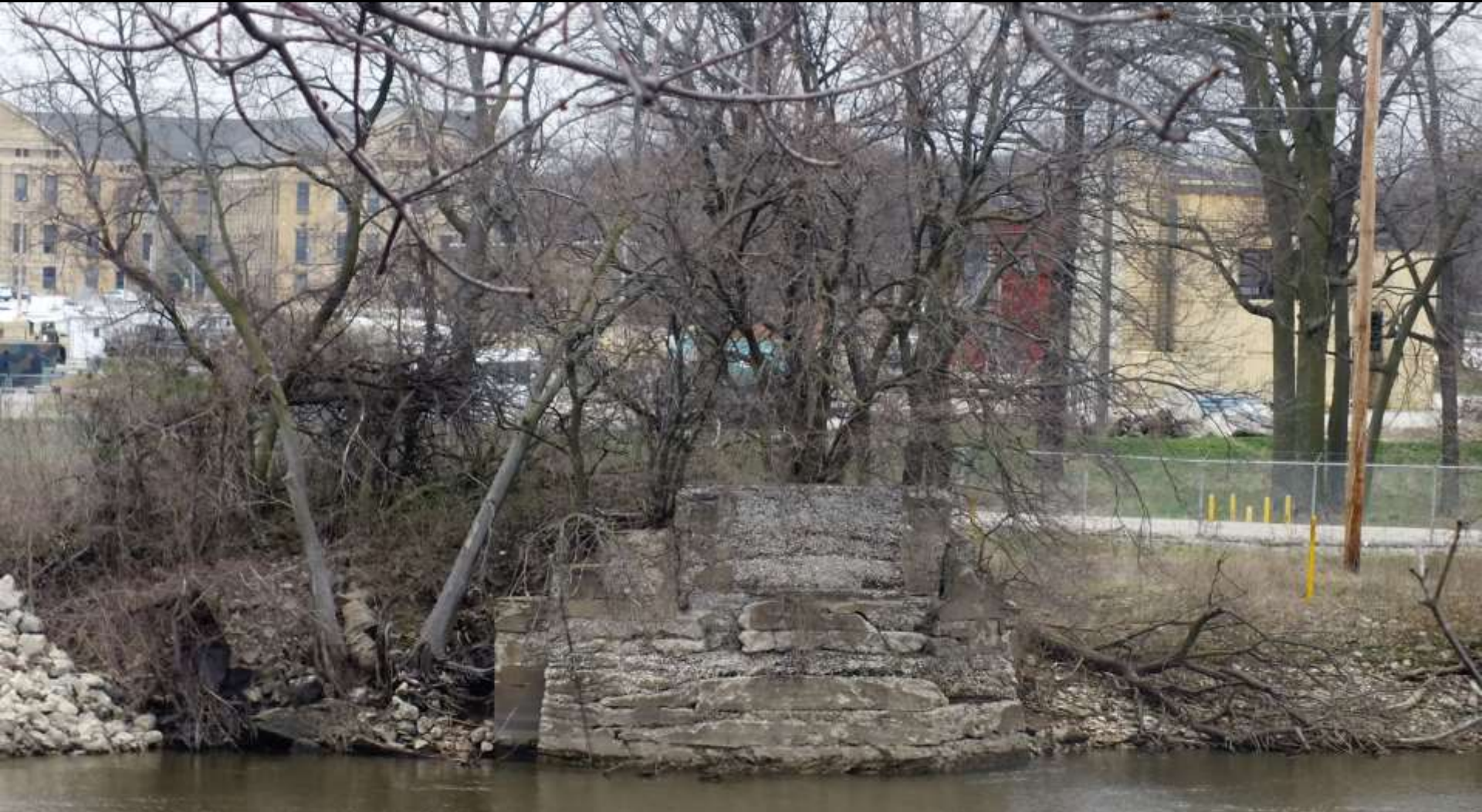
First Bridge at RIA
