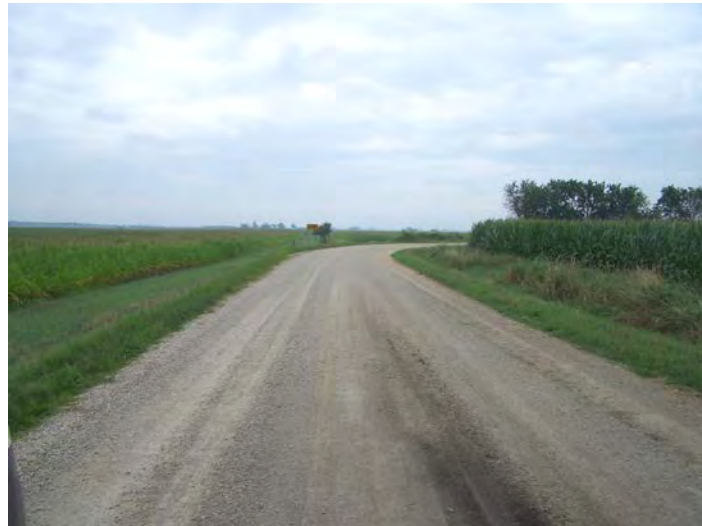
Looking south at curve south of site
