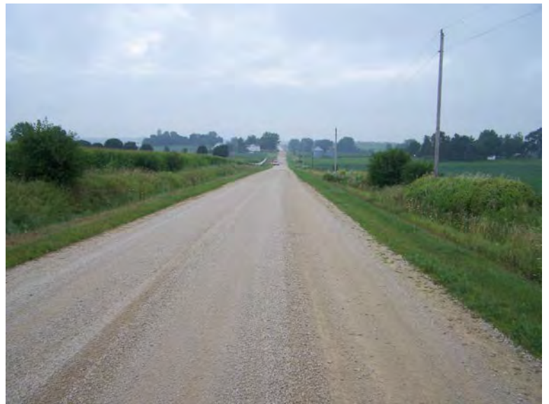
Looking south on 10 th Av north of Mud Creek
