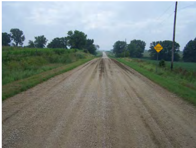
Looking south on 10 th Av north of bridge on Mud Creek
