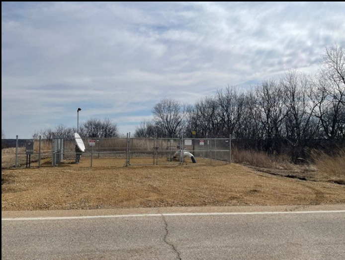
Alliance Pipeline Inc. property, north of subject property
