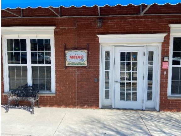
Figure 4.6: LeClaire ADM Station
