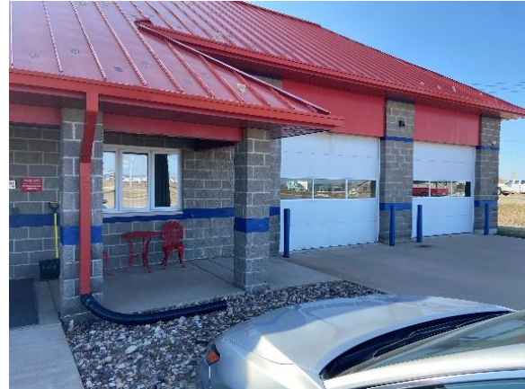
Figure 4.7: Eldridge ADM Station
