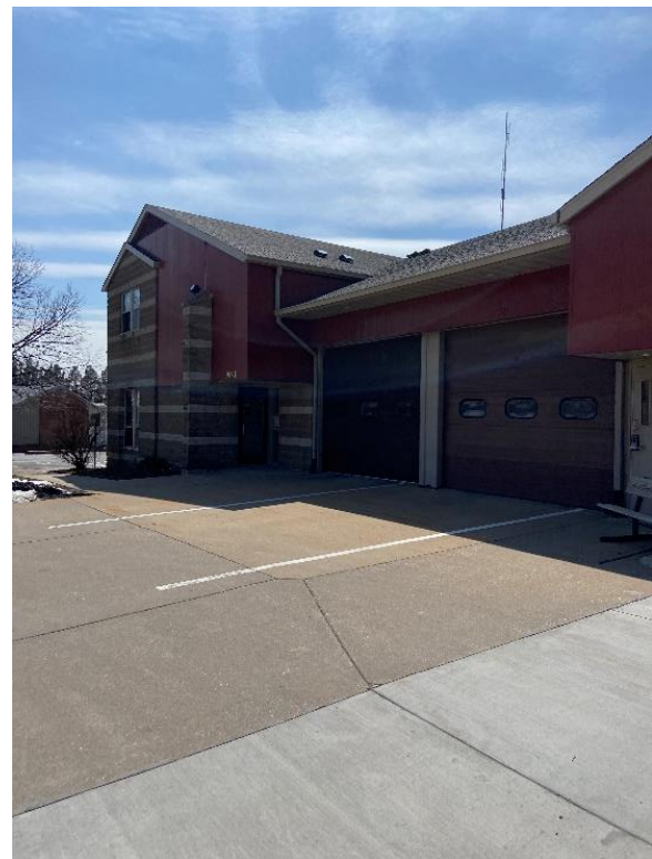
Figure 4.5: Bettendorf Fire Station
