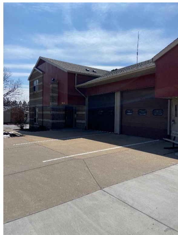
Figure 4.5: Bettendorf Fire Station
